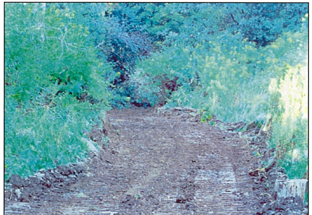
Smoothing ruts in skid trails after use minimizes the channeling and ponding of water during rainfalls and spring melts.
