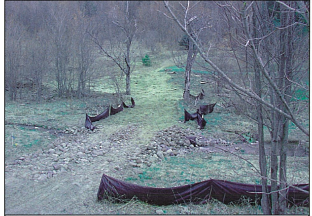
Silt fence is good temporary measure that can be used to capture and prevent sediment from entering a body of water. [Photo courtesy of NYC Watershed Forestry Program]
