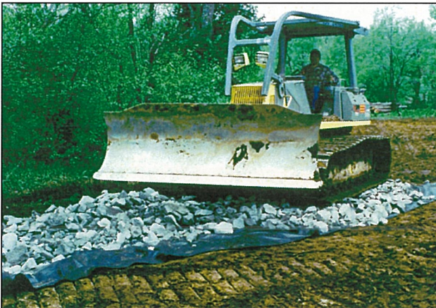
Geotextile mats help stabilize and support forest roads. This material is permeable to water and can help control rutting and water flow.
