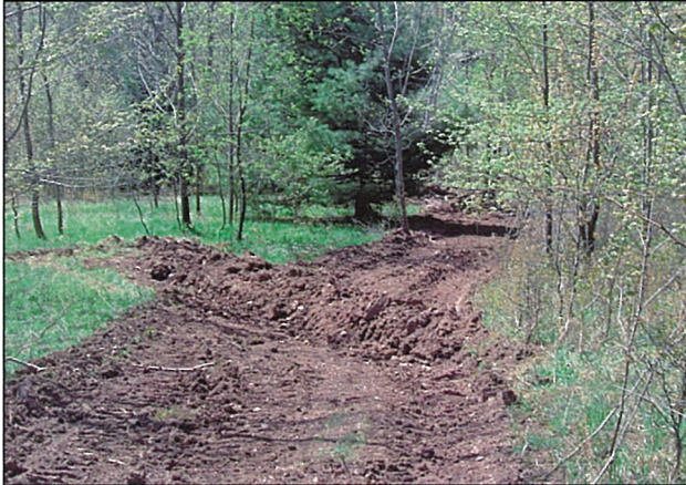
Waterbars are one of the most effective means of slowing and diverting the flow of water off of skid trails, and provides long-term erosion control on slopes. [Photo courtesy of NYC Watershed Forestry Program]
